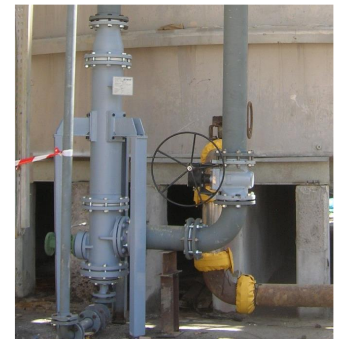
External Diluter with Static Mixer
