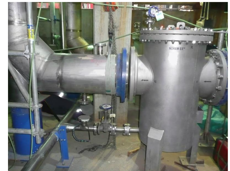
External In-line Acid Strainer Installation
