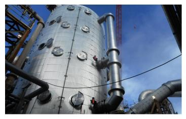
Stainless steel converters using flat bed support plates and divider plates welded to the shell, which basically copy the old carbon steel design, have experienced failures as a result of the differential rate of thermal expansion of the plate and the shell during heat-up.
