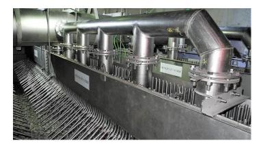
The NORAM Trough Acid Distributor design makes use of evenly spaced downcomer tubes to distribute the acid evenly across the tower cross-section. These downcomers extend into the packing volume directly, reducing acid spray and mist formation, in turn lowering the maintenance costs associated with the tower demisters. The even spacing of the downcomers ensures an even distribution from the trough to the packing.
