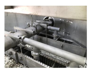
The NORAM Trough Acid Distributor design utilizes assemblies attached to the tower wall for the purpose of post-installation leveling and adjustment. This ensures a very even and stable liquid height in the trough, resulting in equalized flow through all downcomers. With this method, the trough distributor achieves a very uniform distribution.
